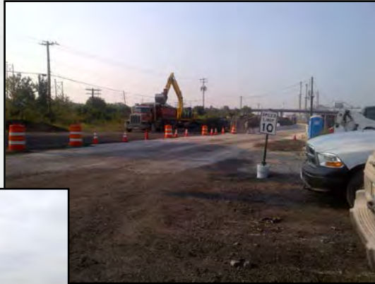
Barrier I Construction
