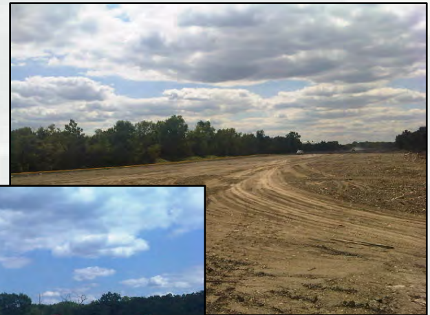
Des Plaines Bypass Improvements
